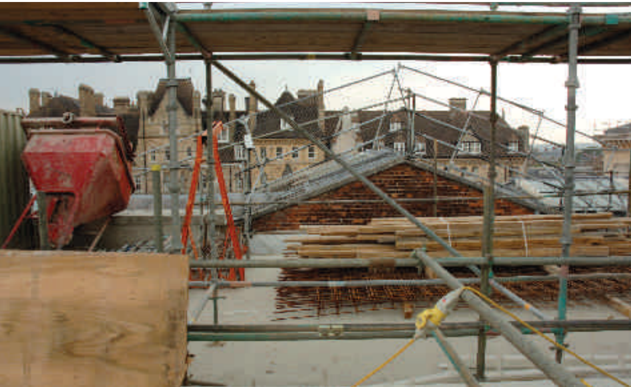
View from the rooftop to the south ▼
