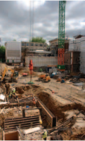
Foundations being laid, May 2007. ▲
