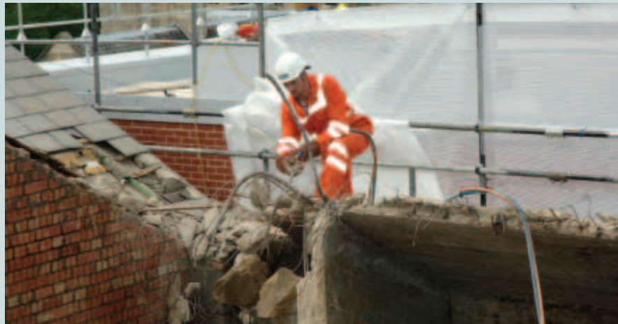
Work underway on the roof of the Drapers' Gallery
